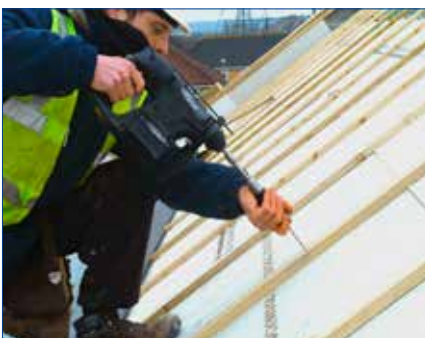
Installing the SureTwist Plus with the Power Support Tool
