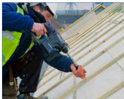
Installing the SureTwist Plus with the Power Support Tool
