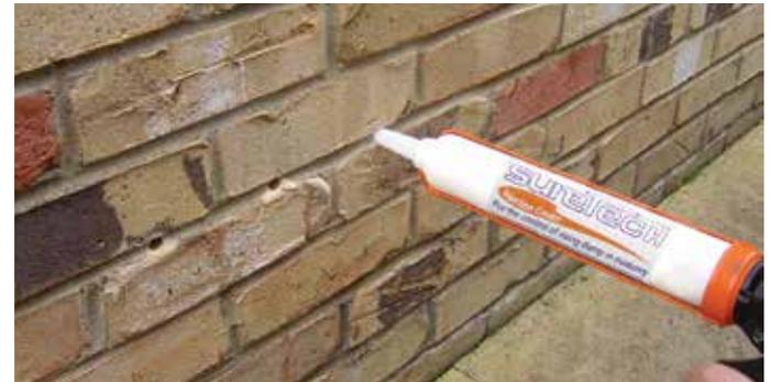
1. 12mm diameter holes drilled horizontally into the mortar joint at 120mm centres and to a depth of 10 - 20mm from the opposite face.
