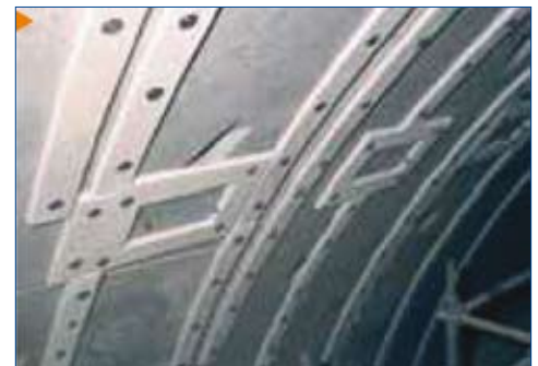
Small SureHit used to attach fire protection board.
