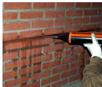
Injecting the bead of grout
