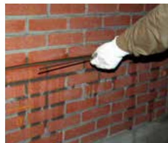
Laying in the bar
